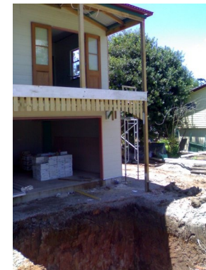
Above: excavation and completion of the in-ground water tank under the driveway in front of the garage.
